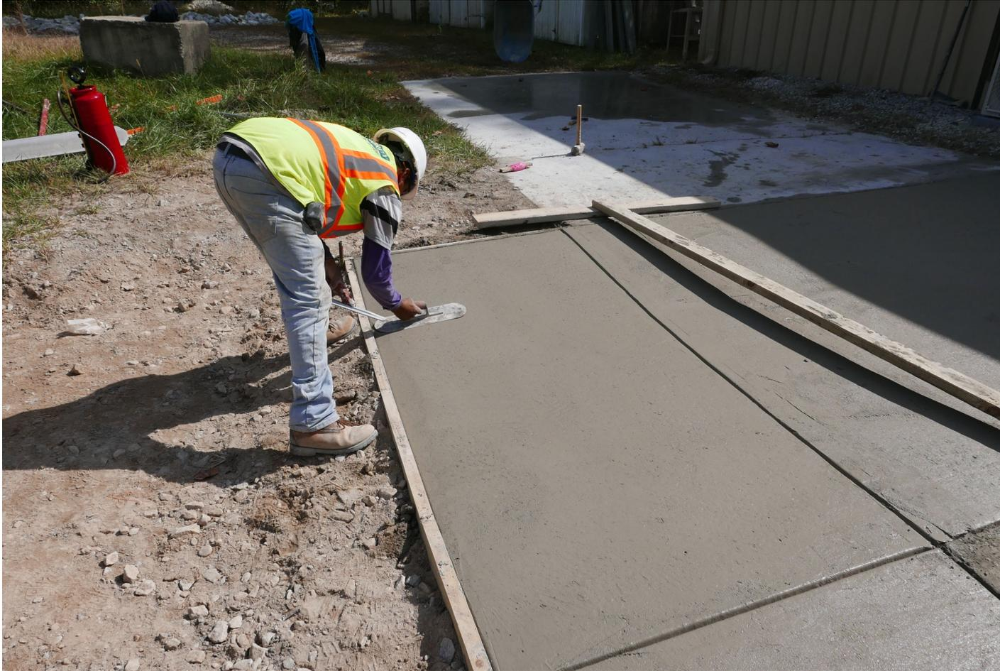
**DO NOT LOAD UP THE BROOM WITH WATER. IT WILL CAUSE THE CONCRETE TO SCALE.**
