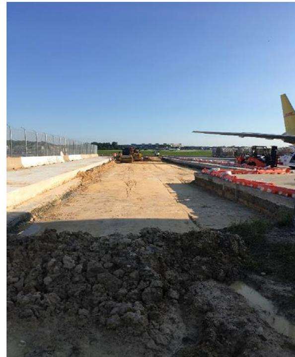
Concrete lane to prevent sheet flow was poured 3 days prior to receiving a half inch of rain in a few short hours.
