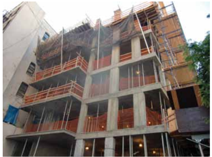
Figure 4. The Vierendeel truss under construction. Courtesy of Jesse Cooper, Severud Associates.
