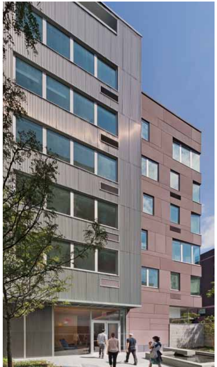
Figure 5. Exterior view of the relaxation garden with the building and the architecturally exposed concrete wall in the background. Courtesy of Eduard Hueber/archphoto.
