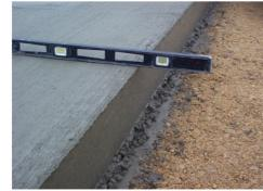
Using a level to check edge slump
