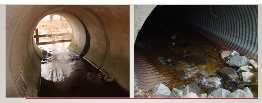
CONCRETE PIPES USUALLY FAIL AT THE JOINTS WHILE METAL PIPES FAIL AT INVERT AS IT RUSTS WHERE WATER IN CONSTANT CONTACT WITH THE METAL.
